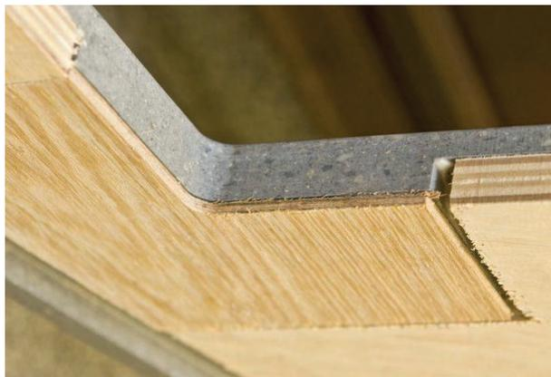
Tube steel, angle iron and wood are acceptable support materials (additional information in Support section). Particleboard and equivalent products are not acceptable as support or underlayment materials. Figures 7, 8, and 9 show support structures of tube steel, angle iron, and wood. In each set of diagrams, Figure A shows support for a cutout corner with the high-strength corner reinforcement block and Figure B shows support for the underlayment between the corner blocks.
